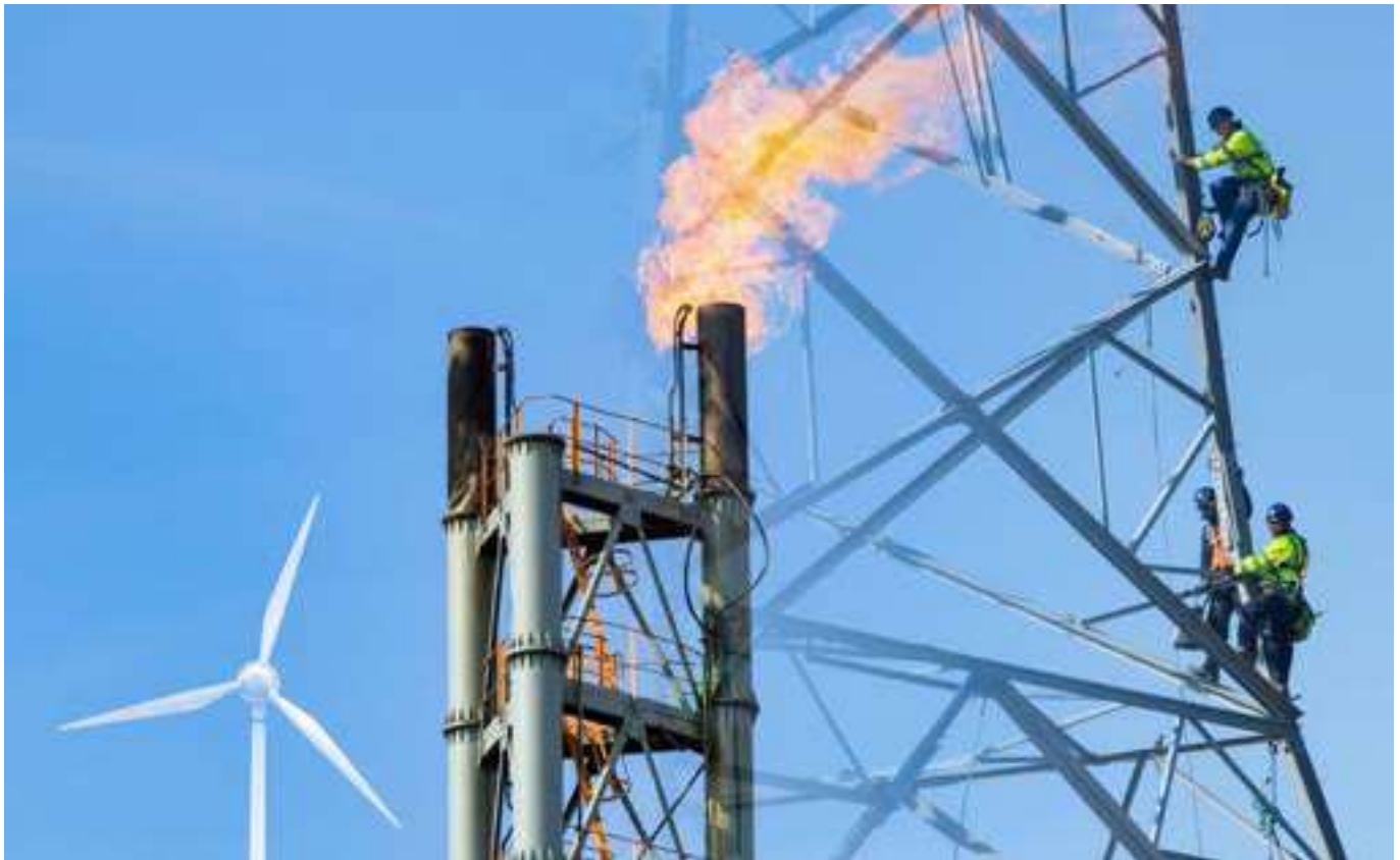
National Grid gas distribution operations
