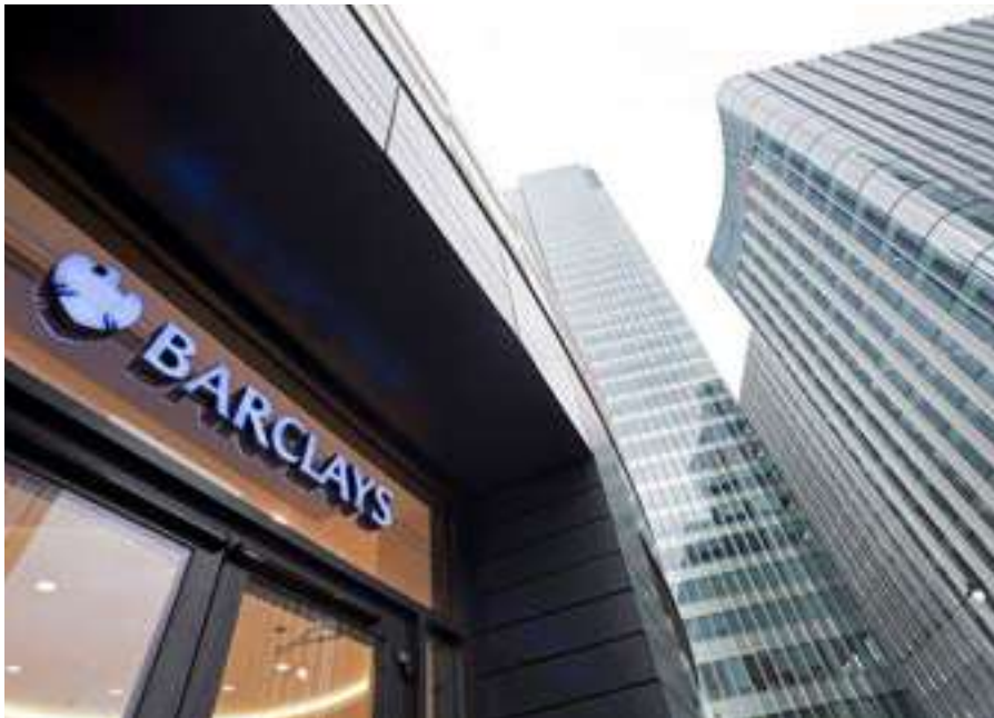
Headquarters of Barclays Bank in Canary Wharf
